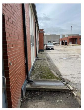
Curb and gravel in this picture removed and just take the new driveway concrete to the building wall with an expansion board. This area is about 3' wide from the building out to the pavement.
