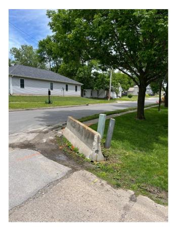
Picture showing the east side where 6" straight back curb will have to transition to a depressed curb at the sidewalk. Crossing of the sidewalk needs to be ADA compliant. Around the yellow mark on the driveway is where an angle at 45 degrees can be made to Vine Street to tie 6" straight back curb into the Vine Street curb.
