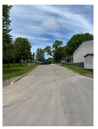
Picture showing the entrance from Vine Street into MMU Facility. Along the west and east sides where the yard is located, the driveway needs to have 6" straight back curb and gutter. 69' on the east and 79' on the west. This pictures also shows the section that will be widened to 32' including the gutters.
