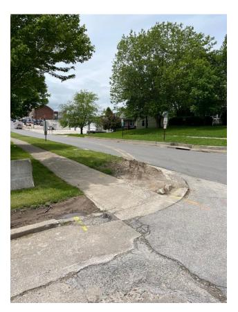
Picture showing the west side where 6" straight back curb will have to transition to a depressed curb at the sidewalk on the west side. Crossing the sidewalk needs to be ADA compliant.
